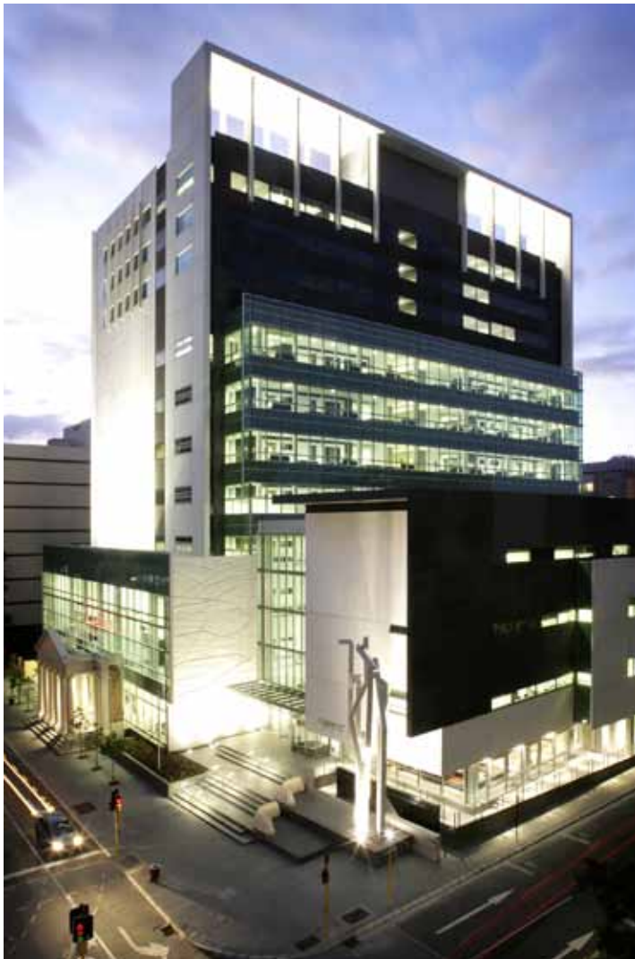
The District Court Building in the heart of Perth.
