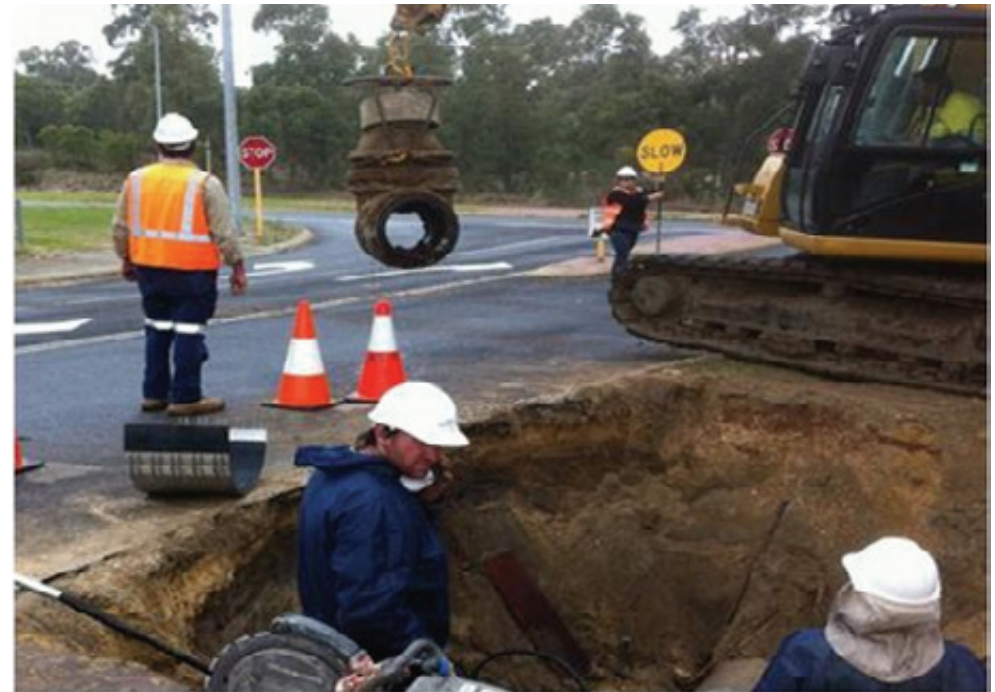
Removing the 450 mm trunk main valve on Underwood Street after 41 years of service.
