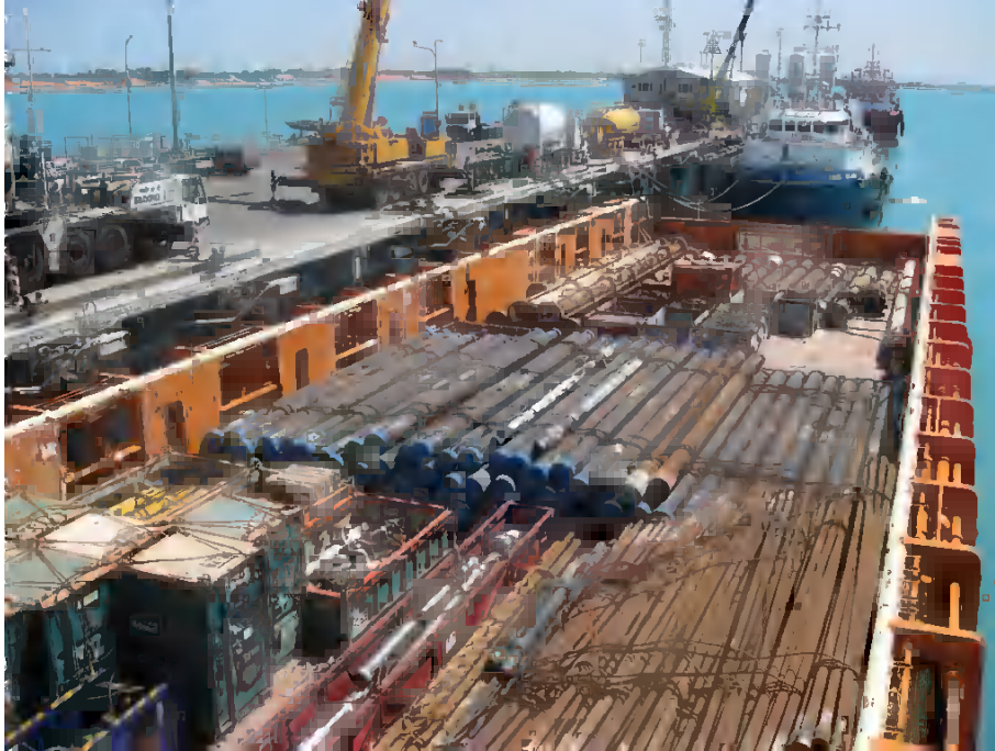
Figure 13 – Drilling equipment loaded on a large rig tender using BrPA cranes
