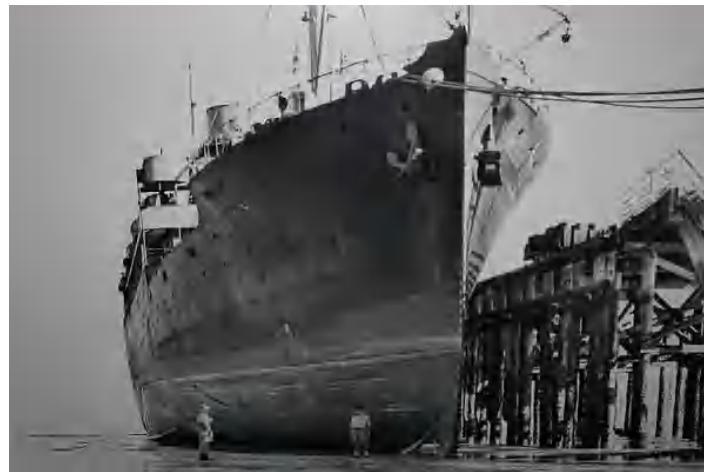
Figure 4 – The original wharf provided a NAABSA 'not always afloat but safely aground' berth.
