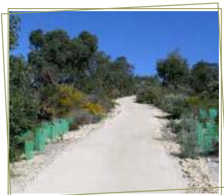
The track upgrade project at Bold Park provides an improved walking surface and better drainage. Photo: B Fellows
