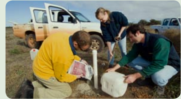
Installing a piezometer to monitor ground water.
