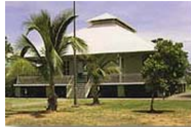
Broome Courthouse, originally Cable House constructed by the Eastern Extension & China Telegraph Co. - 1890's.
