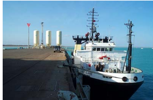
Dry bulk storage silos installed for oil and gas industry – with Rig Tender Lady Elaine alongside
