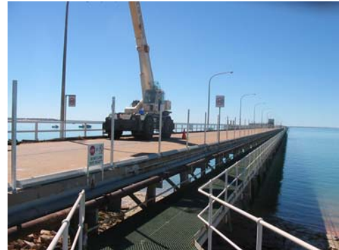
New security fence along boardwalk under construction during June 2004
