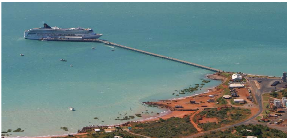
Broome Port – 700m long neck to serve vessels at 183m long berth – Superstar Virgo alongside
